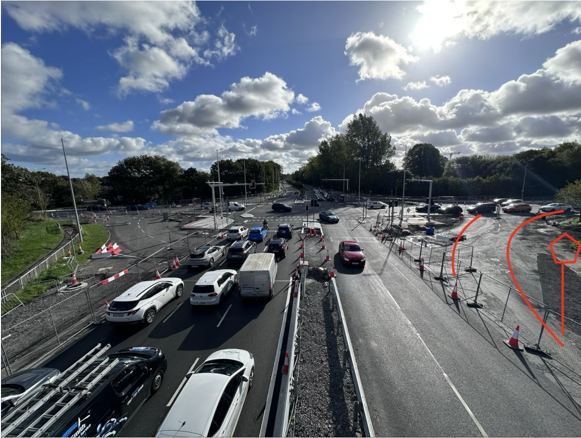
Figure 2. Live view of the Estuary junction during current works. The red annotation shows the same potential temporary slip route and stop controlled merge point in the existing physical space.
